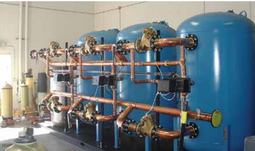
System shown with optional ProPress plumbing.
